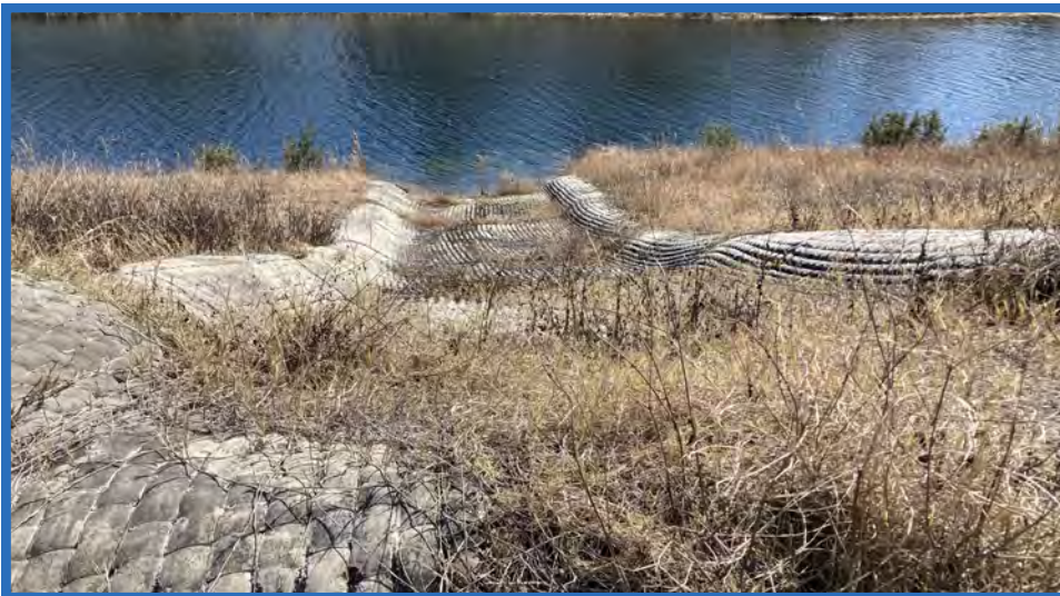
Fabriform-Lined Flume from Southern Part of Eastern Containment Dike of Stage I into Stormwater Pond B, Looking East
