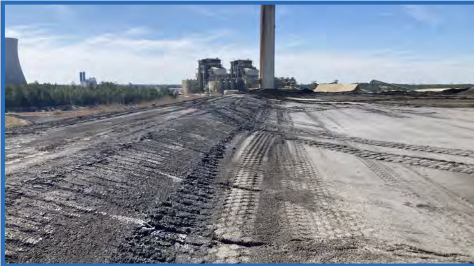
Top of Waste in Stage I, Looking Southwest
