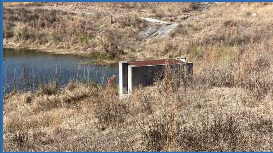
Outlet Structure CS-1 for Stormwater Pond B, Looking West from Perimeter Road Around Eastern Side of Pond B
