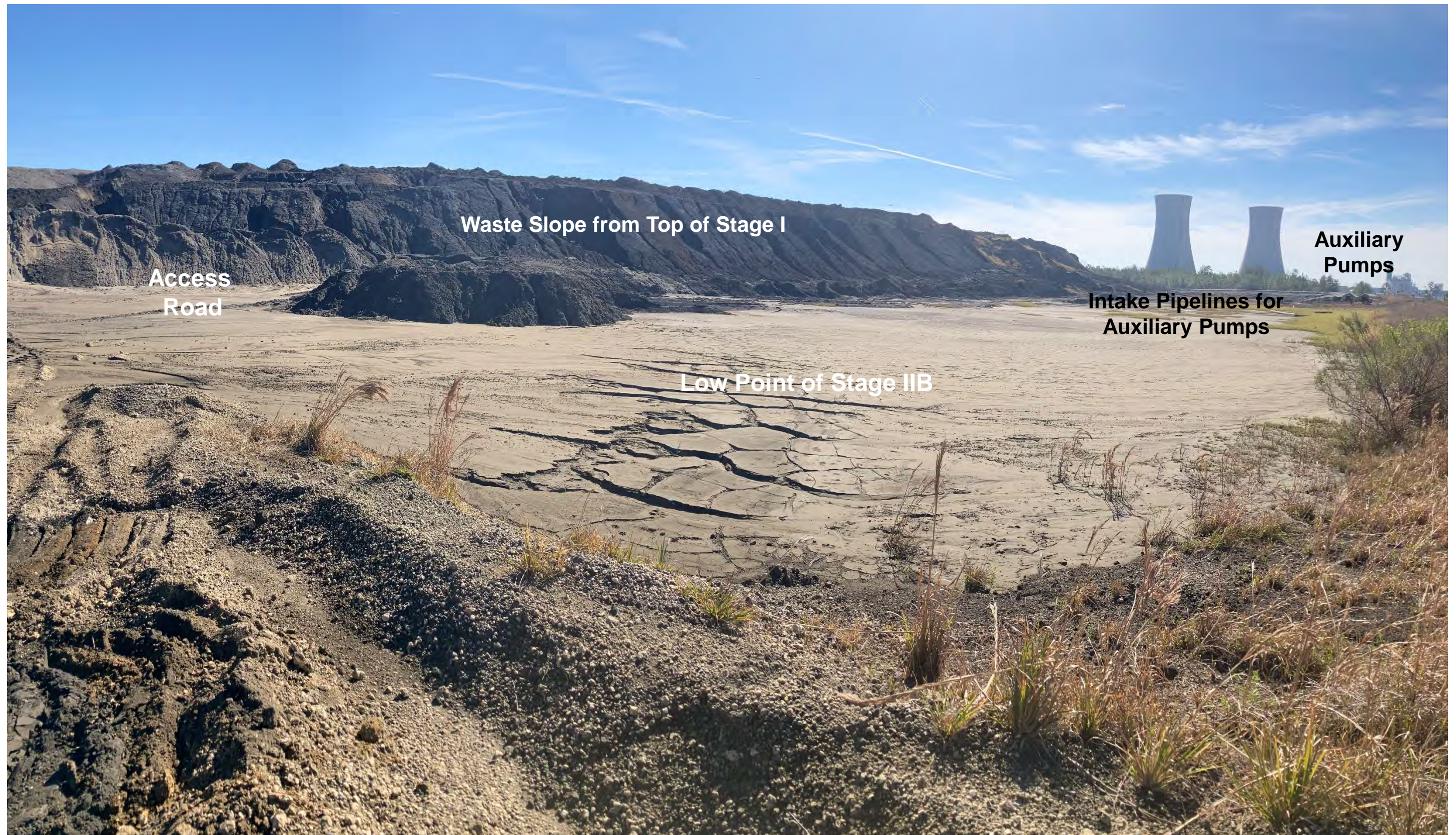
Low Point of Stage IIB, Looking Southeast
