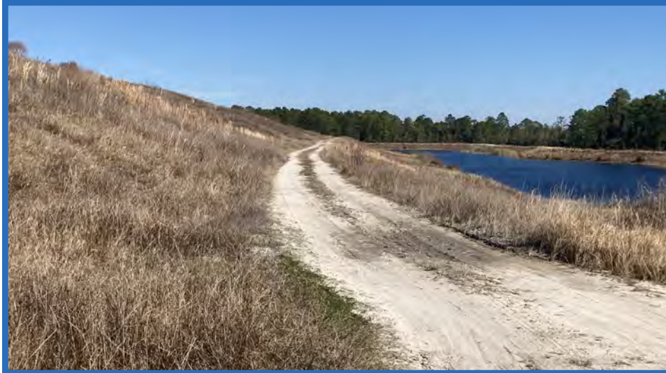
Perimeter Road, Eastern Slope of Containment Dike for Stage I, and Stormwater Pond B, Looking North
