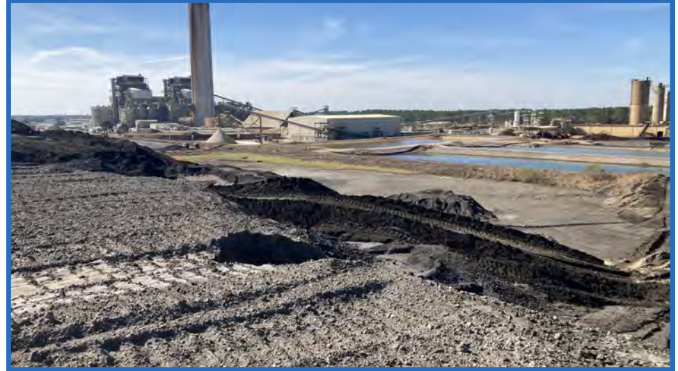
Stage IIB, Looking Southwest from Top of Stage I
