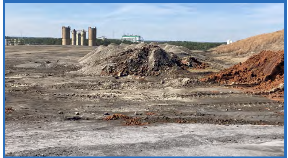
Piles of Fly Ash and Dewatered PWT Sludge on Top of Stage I, Looking West
