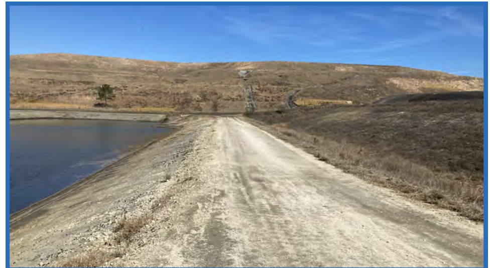
Perimeter Road and Swale Along Toe of Western Containment Dike for Stage IIB, Looking North Toward Closed Original Landfill and Vertical Expansion
