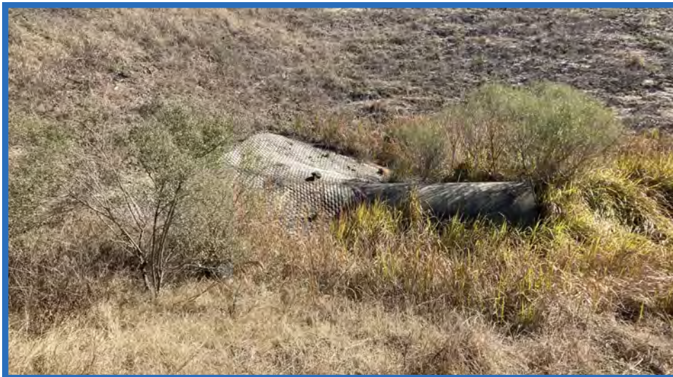
Fabriform Around Reinforced Concrete Pipe Under Access Ramp to Stage IIB, Looking East
