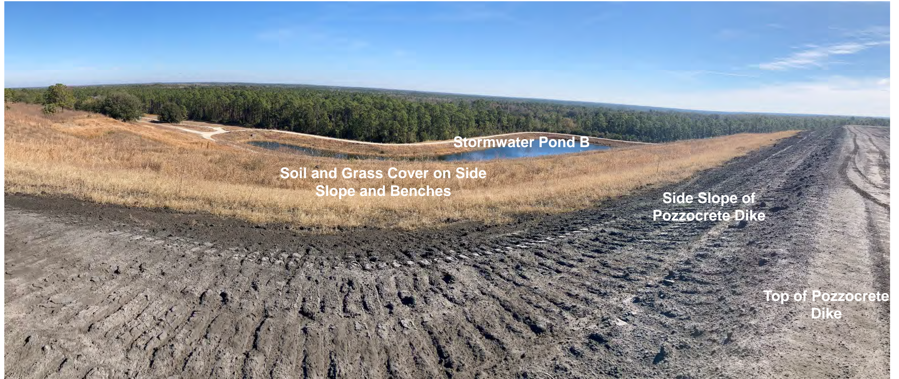
Pozzocrete Dikes, Side Slopes, and Benches on Eastern Side of Increment 1, Stage I, Looking East Toward Stormwater Pond B
