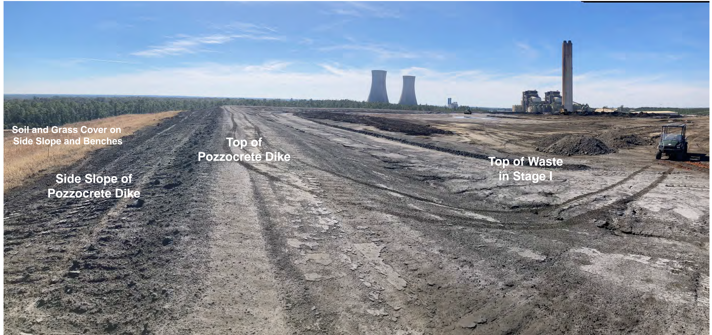
Top of Increment 1, Stage I, Looking South
