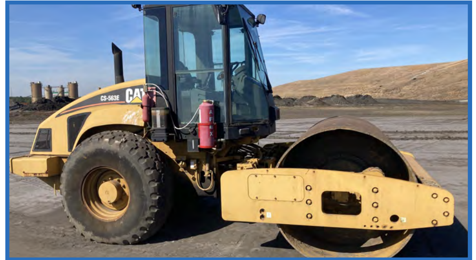
Caterpillar 563C Compactor on Top of Stage I
