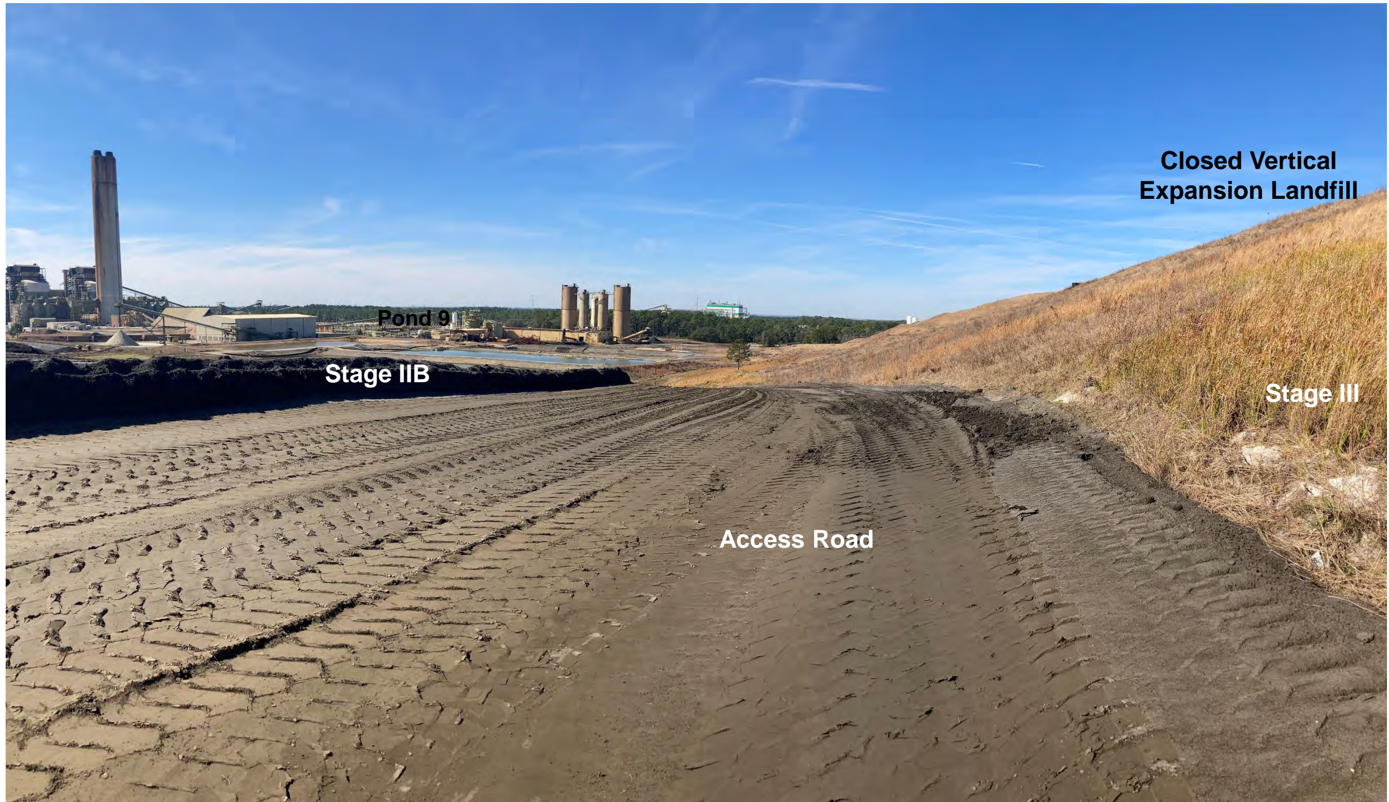
Access Road to Top of Stage I and Stage III, Looking Downhill to the West
