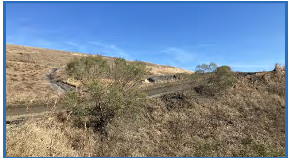
Access Ramp to Stage IIB, Looking Northeast
