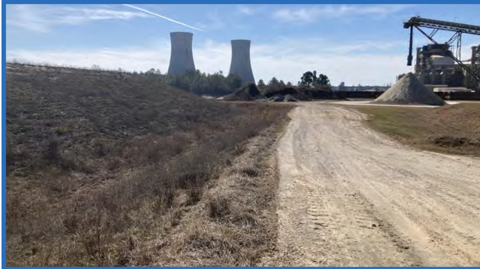
Containment Dike for Stage IIB, Perimeter Swale and, Perimeter Road, Looking South
