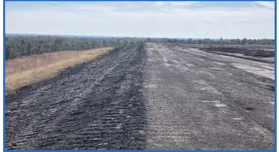
Pozzocrete Dike at Top of Waste on Eastern Side of Stage I, Looking South Along Dike
