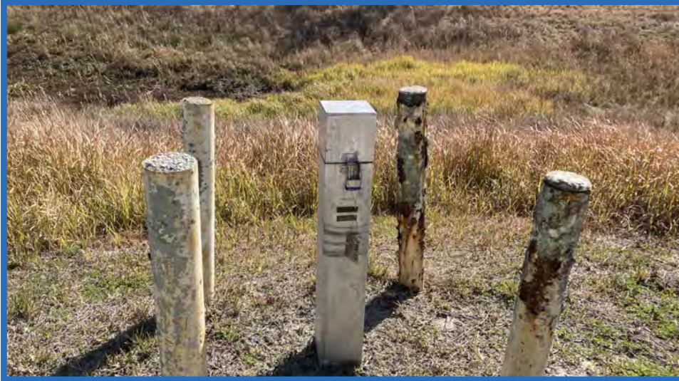
Monitor Well MW-19, Looking East Toward Culvert Outlet into Stormwater Pond B
