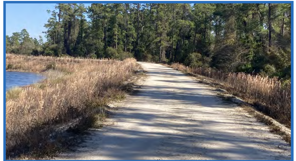
Perimeter Road Around Eastern Side of Pond B, Looking North
