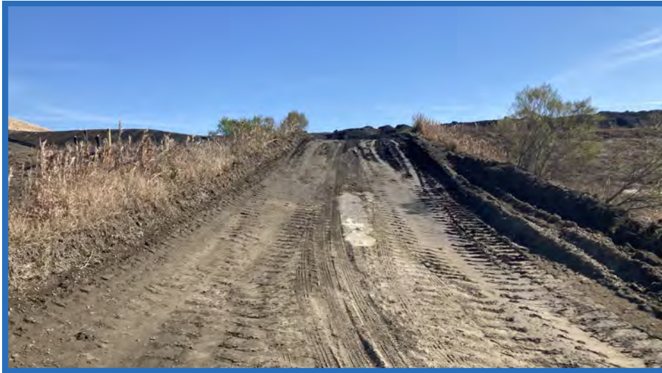
Access Ramp to Stage IIB, Looking East
