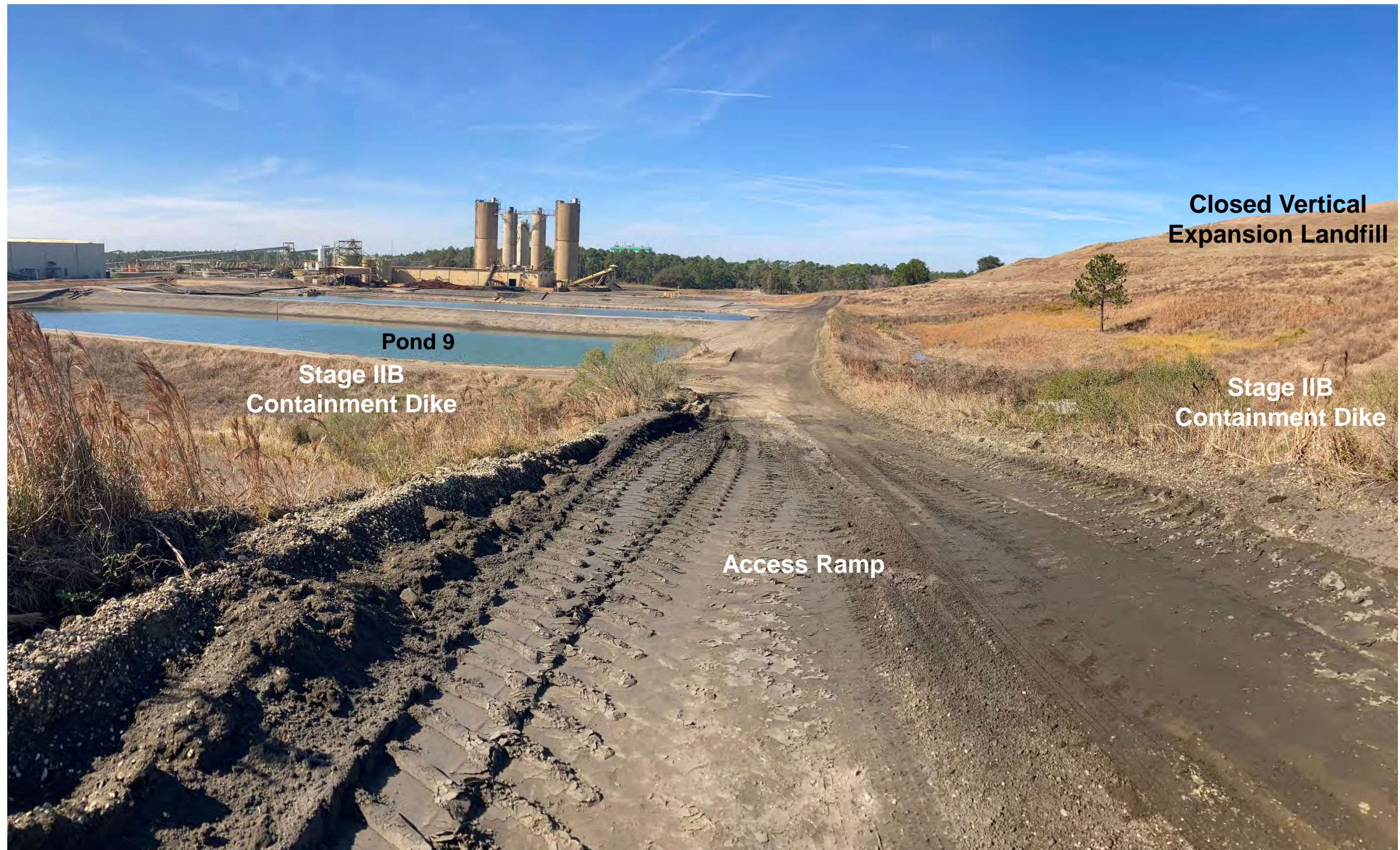
Access Ramp to Stage IIB, Looking Downhill to the West
