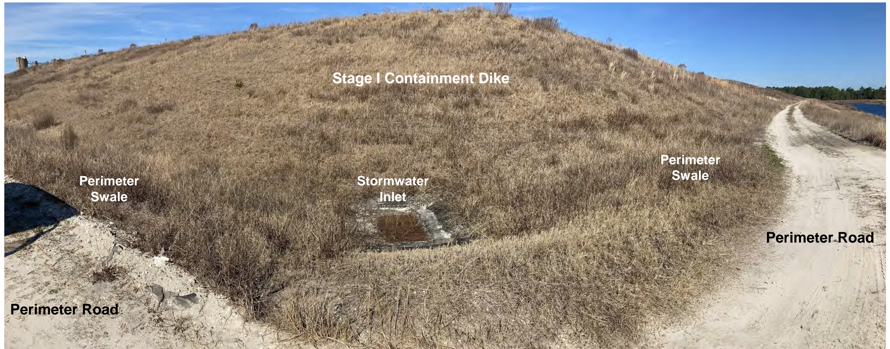
Stormwater Inlet in Perimeter Swale at Southeastern Corner of Stage I Containment Dike, Looking Northwest
