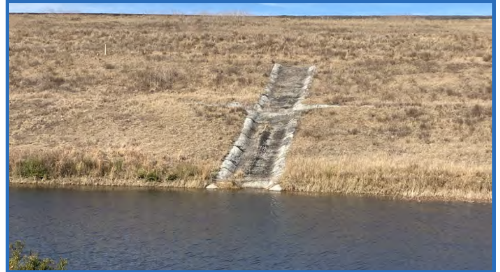
Eastern Slope of Increment 1 and Fabriform-Lined Flume into Stormwater Pond B, Looking West from Perimeter Road Around Eastern Side of Pond B
