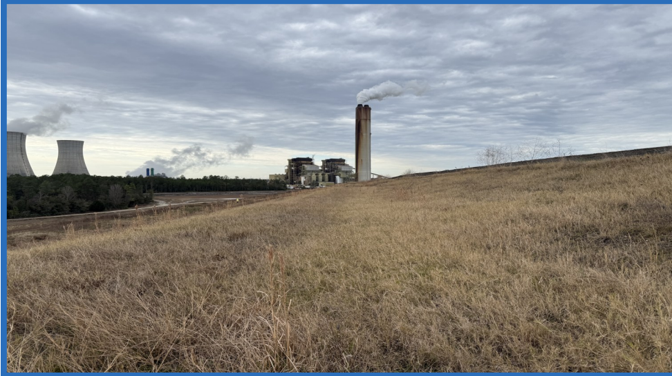
Covered Pozzocrete Slope on South Side of Increment 1 (Looking West)
