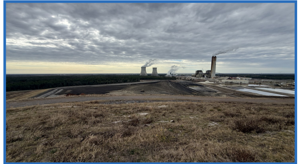
Increment 1 from Top of Vertical Expansion (Looking South)
