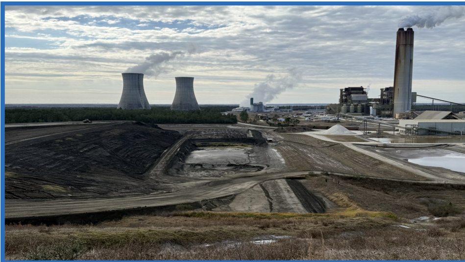
West Side of Increment 1 (From Top of Vertical Expansion Looking South)
