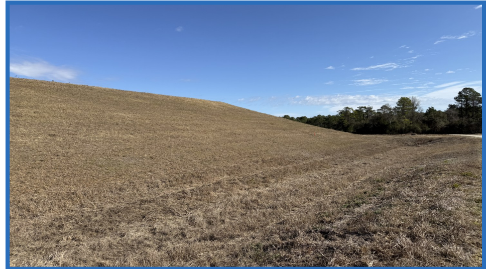
South Containment Dike of Increment 1 (Looking East)
