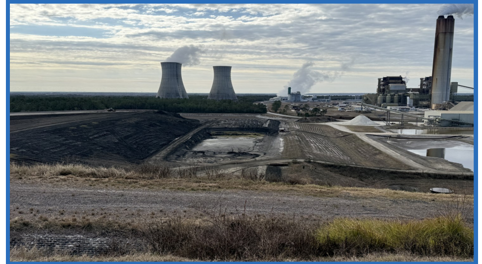
West Side of Increment 1 (From Top of Vertical Expansion Looking South)
