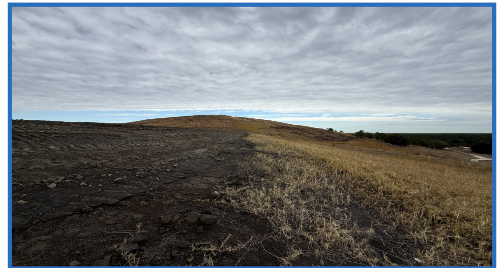
Pozzocrete Dike on East Side of Increment 1 (Looking North)
