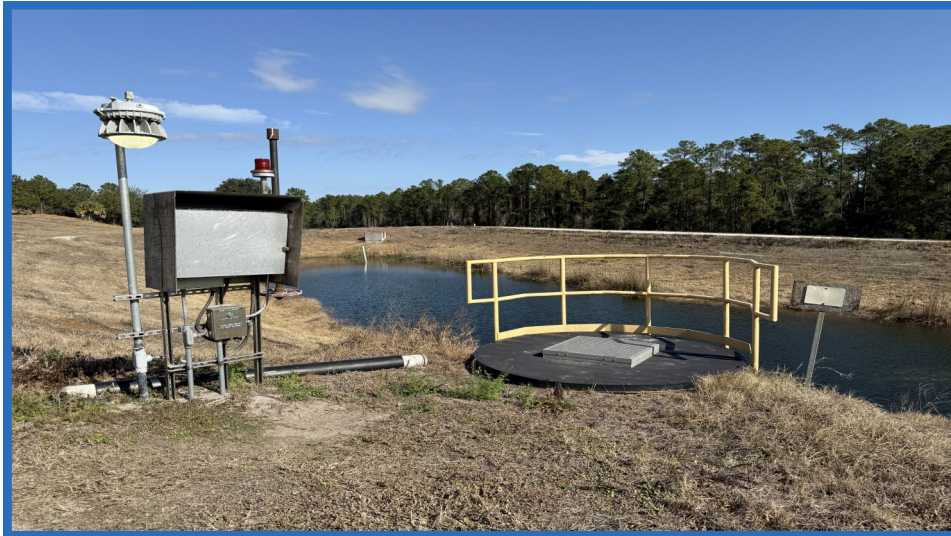
Increment 1 Leachate Pump Station (Looking Northeast)
