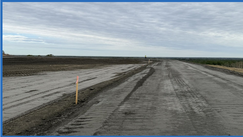
Pozzocrete Dike on South Side of Increment 1 (Looking East)
