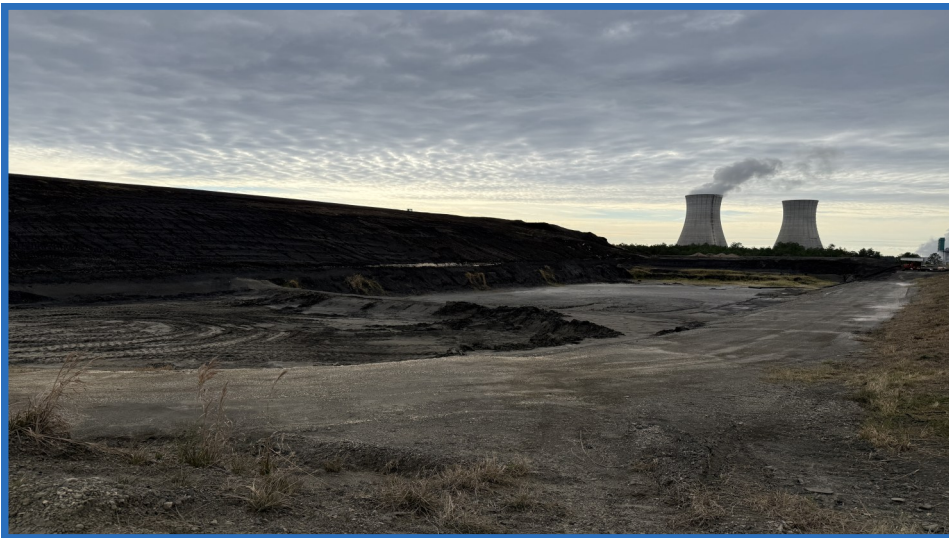
Low Area on West Side of Increment 1 (Looking South)
