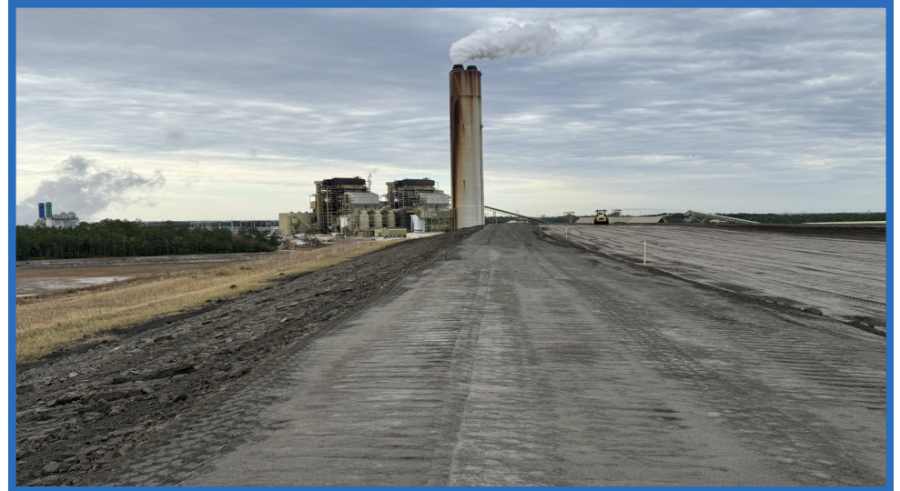
Pozzocrete Dike on South Side of Increment 1 (Looking West)
