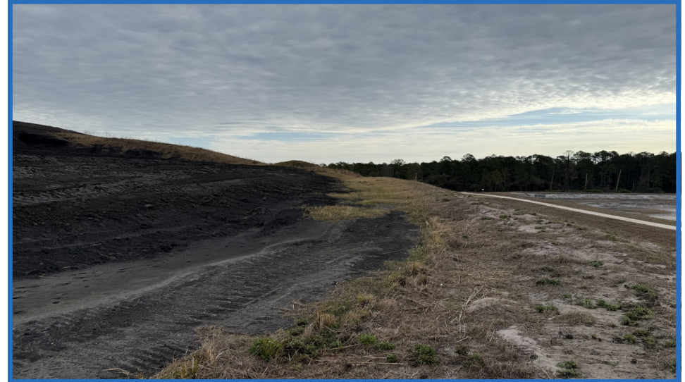
Pozzocrete Slope on South Side of Increment 1 (Looking East)
