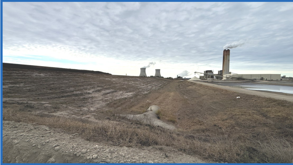
Containment Dike Slope on West Side of Increment 1 (Looking South)
