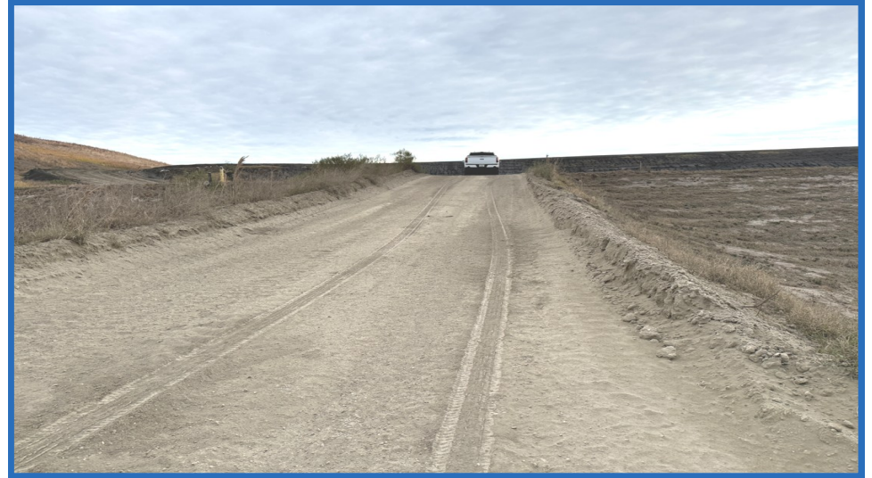
Access Ramp into Increment 1 (Looking East)
