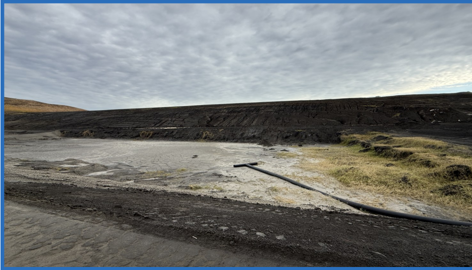
Auxiliary Pump Intake on West Side of Increment 1 (Looking Northeast)
