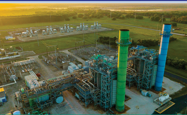
Midulla Generating Station (MGS) Hardee County, FL
