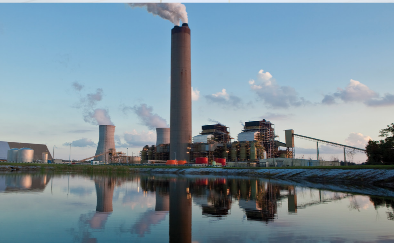
Seminole Generating Station (SGS) Putnam County, FL
