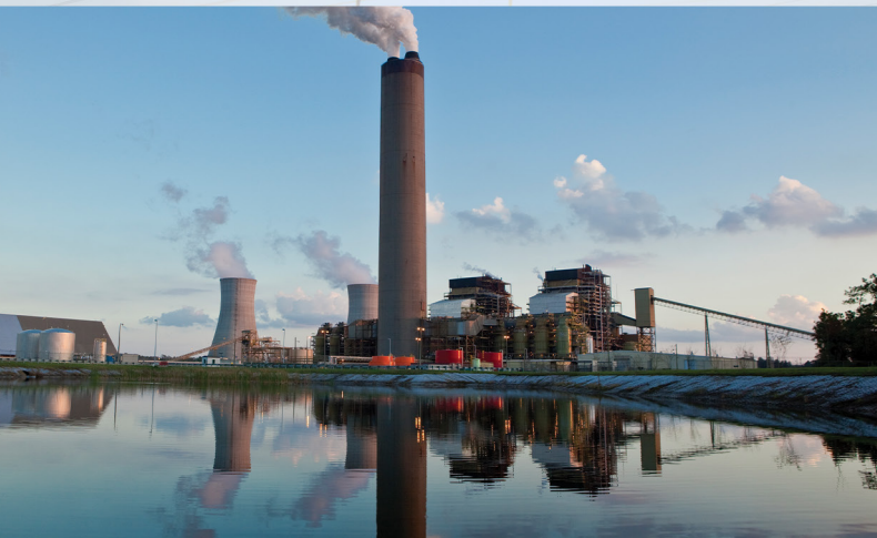
Seminole Generating Station (SGS) Putnam County, FL
