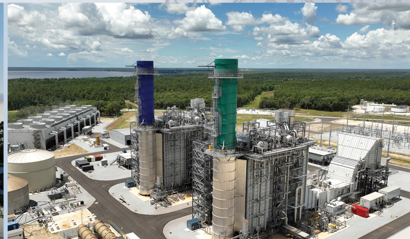
Seminole Combined Cycle Facility (SCCF) Putnam County, FL
