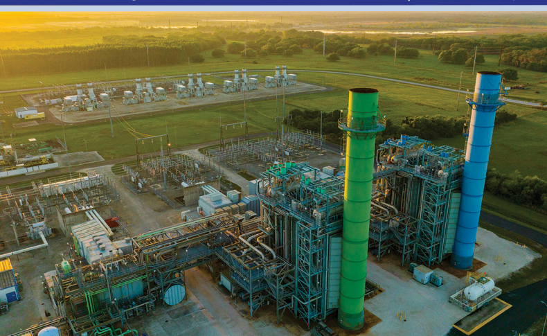
Midulla Generating Station (MGS) Hardee County, FL
